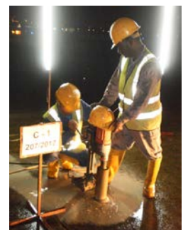
Coring to inspect the construction materials
